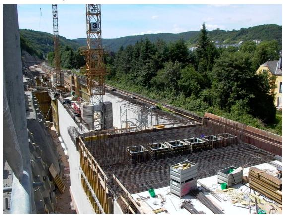
Heat and smoke exhaust units will be placed across the tunnel roof at right angles to the tunnel axis. In this way all heat and smoke released from a car fire can be removed best. A separate ventilation system with jet fans will be provided for the control of the air pollution inside and outside of the tunnel (09. June 2003).
