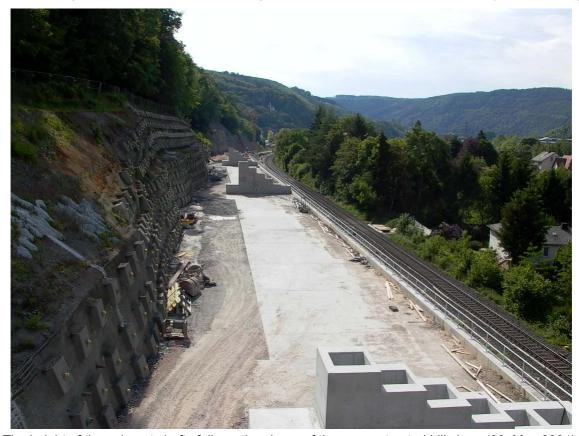
The height of the exhaust shafts follows the shape of the re-constructed hill slope (20. May 2004).
