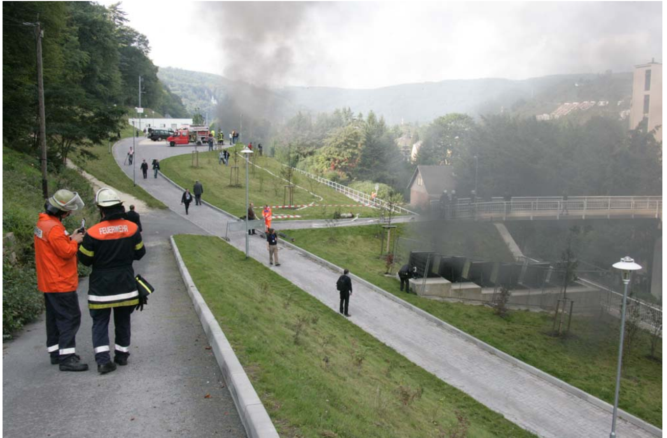
Picture 33: The clouds of smoke were discharged from the smoke exhaust shafts #05 and #06 (both were at nearest to the fire place), viewed after 22 minutes from the east.
