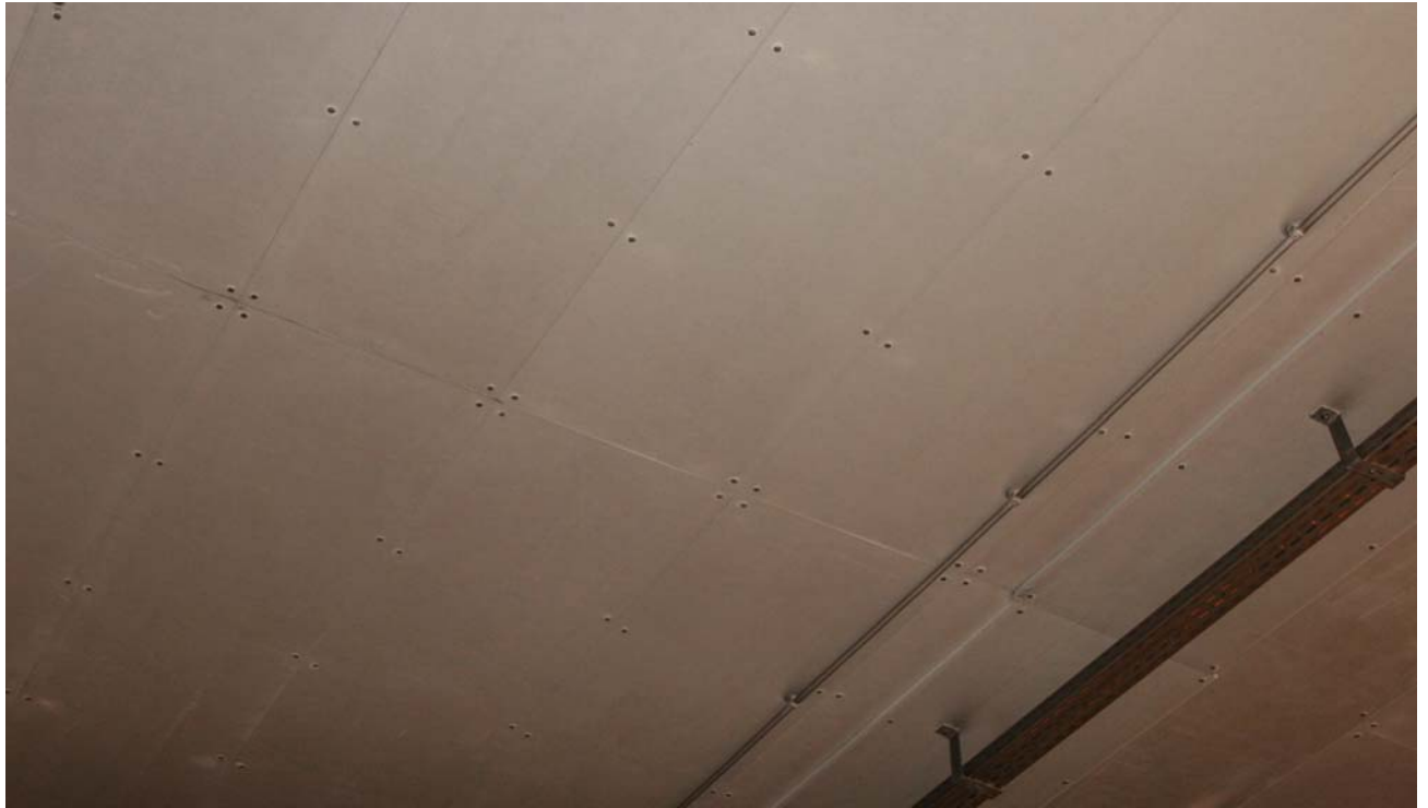
Picture 22: The heat protection at the ceiling, 9.5 m wide, 100 m long, made of 15 mm heat retardant plates. The light fittings, fire detection cable, radio antenna, electric cables, loud speakers, CCTV-cameras and measuring instruments remained unprotected, except the encapsulated ultra-sonic meters.
