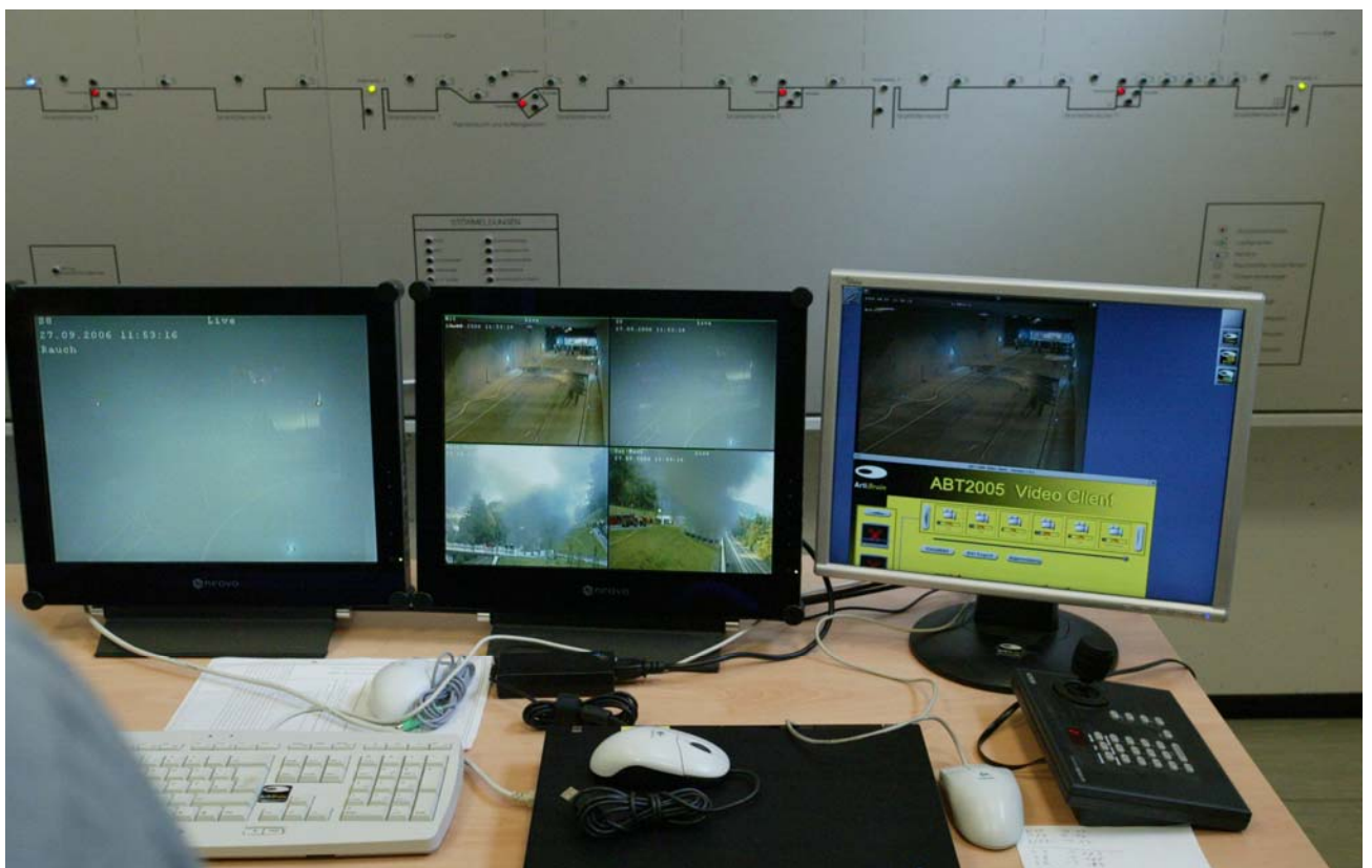
Picture 46: The control room has been furnished with a mimic board on the wall for the indication of the condition of the lighting, ventilation, smoke extraction, alarms, failures and traffic congestions. Video monitors have been placed on the desk next to the process monitors to supervise the traffic flow. Due to the dark smoke the video cameras and monitors went blind and were of no use during the test.
