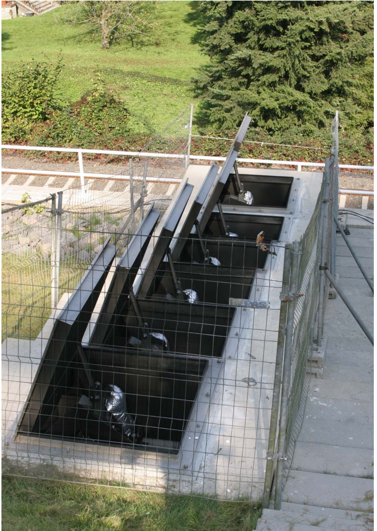
Picture 51: The dampers of the smoke extracting station remained unharmed and have been well functioning after the test (this was the station #06 with dampers, levers and heat insulated gear motors).
