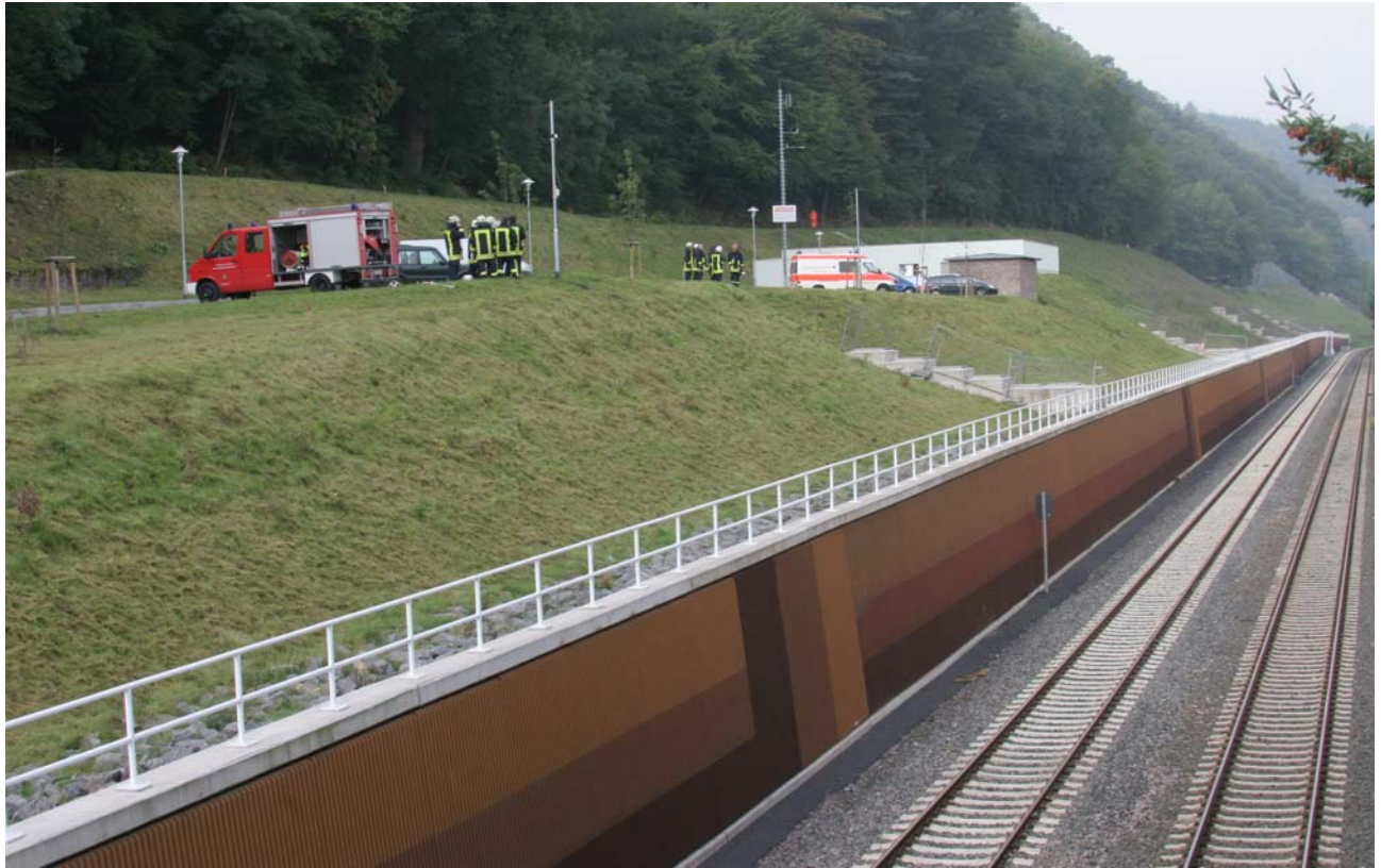
Picture 18: The site of the control building and of one, out of six, emergency stair-cases, and of five smoke extracting stations, out of twelve, located at the foot of the northern “Malberg” hill side.
